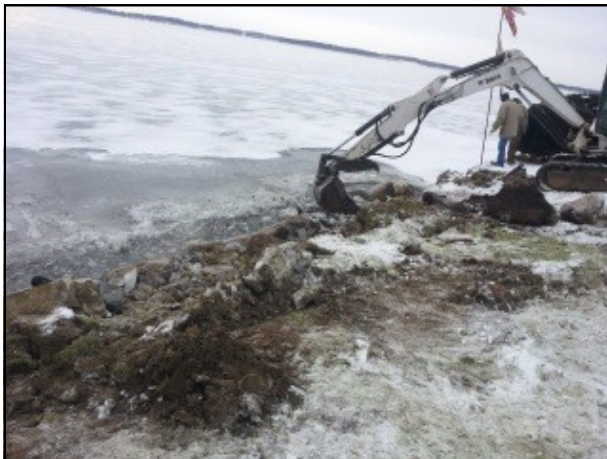
Lake Monona shoreline before restoration. Photo credit: David Bohl
